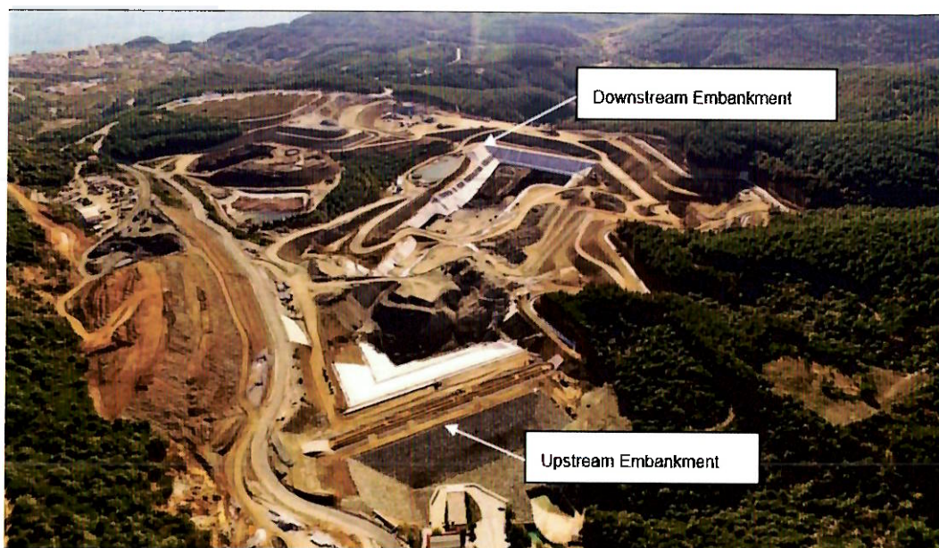
Figure 5-2: Photograph of Kokkinolakkas WMF during Construction (Looking Southeast)
