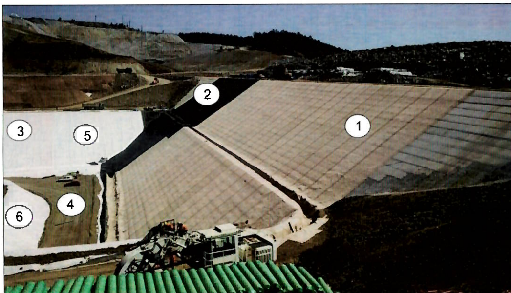
Figure 5-8: Composite Liner System
