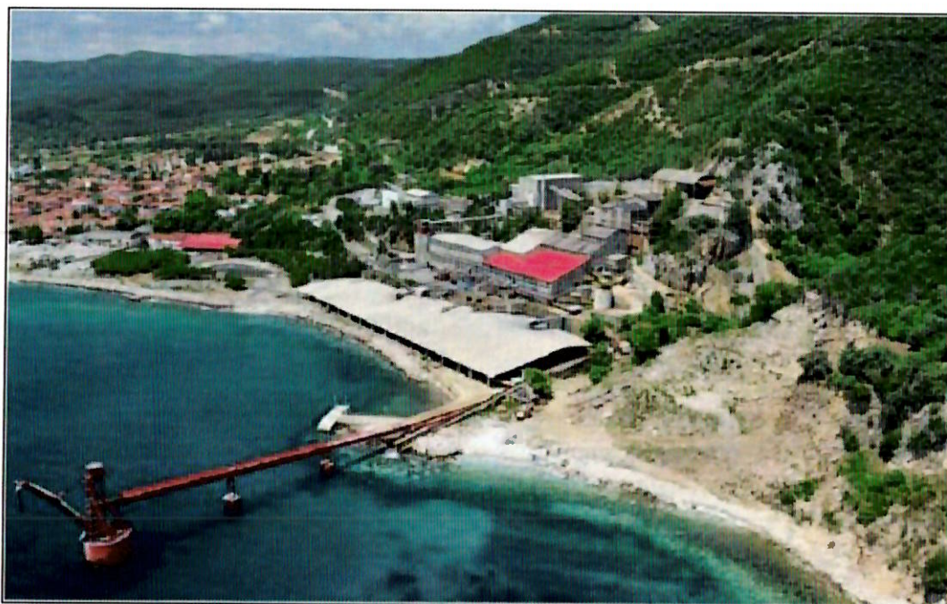
Figure 6-2: Stratoni Port: Existing Infrastructure
